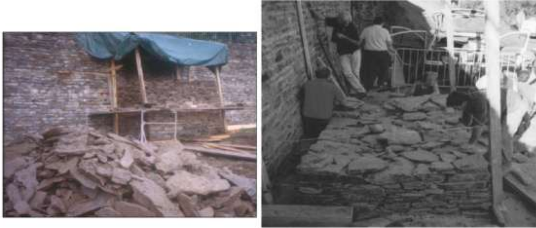
Fig. 5. Wall 5 construction; left: stone size heterogeneity, right: wall basement construction.
